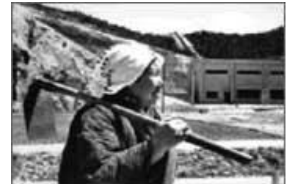
Public Water Project in Aichi Prefecture: 1957
