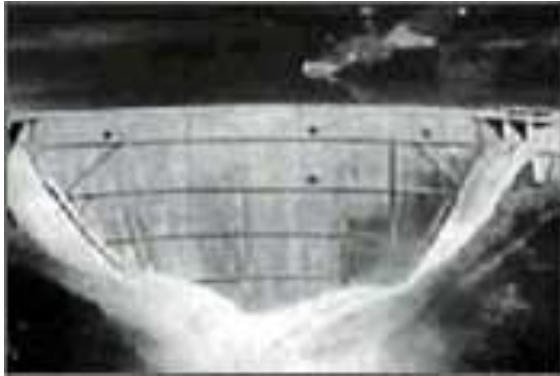
Kurobe No.4 Hydroelectric Power Station: 1964
