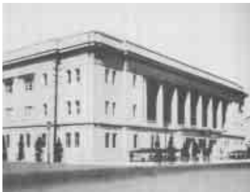
The headquarters of the Bank of Taiwan.
