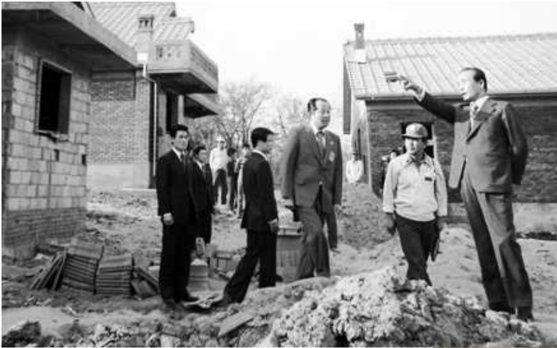
President Park visiting a rural housing construction site
