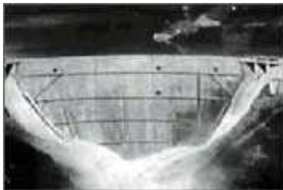
Kurobe No.4 Hydroelectric Power Station: 1964
