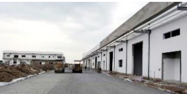
Vie-Pan under construction (Sep.2014)
