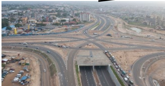
The Tema Motorway Interchange (Ghana)
