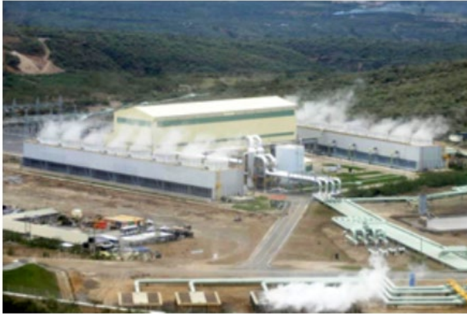
Geothermal in Kenya (Photo: Toyota Tsusho)
