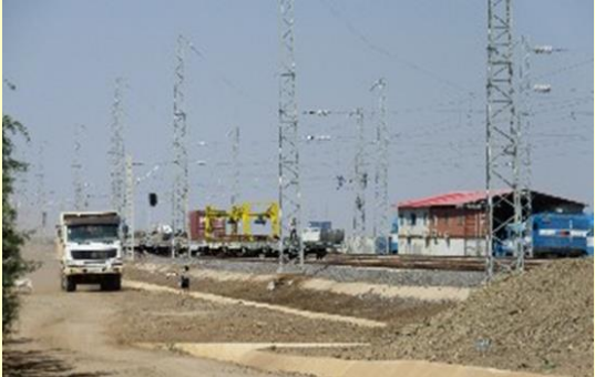
Addis-Djibouti New Railway under construction
