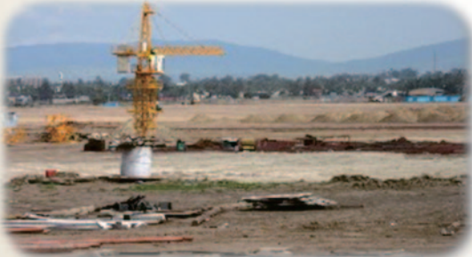
Constructing Hawassa Industrial Zone
