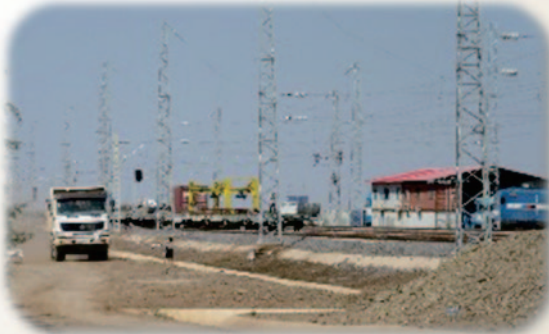
Addis-Djibouti New Railway under construction
