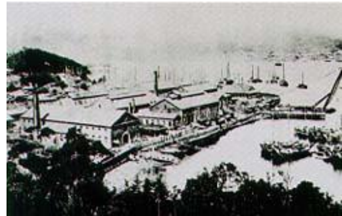
Mechanical factory in Nagasaki, ca 1885
