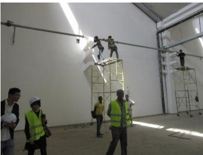
Pipe installation work inside a shed
