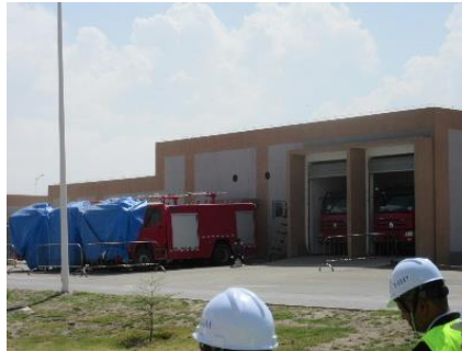
Fire station and fire engines covered with blue sheets
