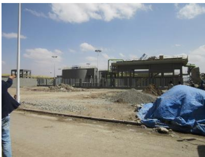
Debris left on the road
