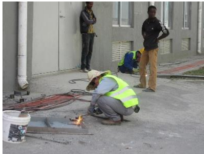
Welding outside a shed
