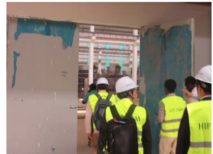
Blue protection sheets must be removed completely
