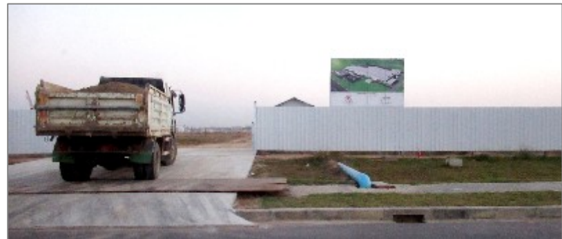
Toyota Myanmar plant under construction
