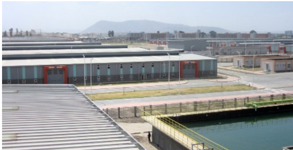
Hawassa Industrial Park
