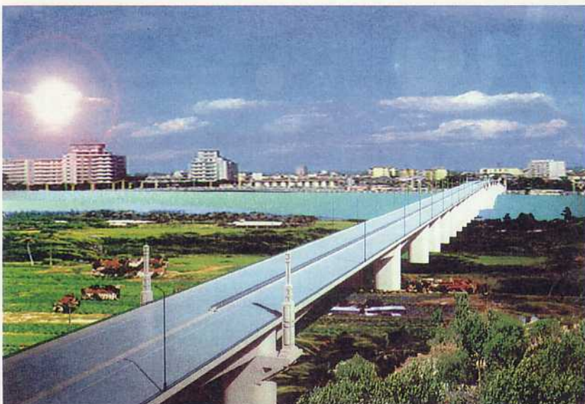
Red River Bridge in Ha Noi financed by JBIC (Image Photo)
