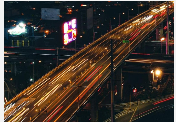
Metro Manila Skyway Stage 3
