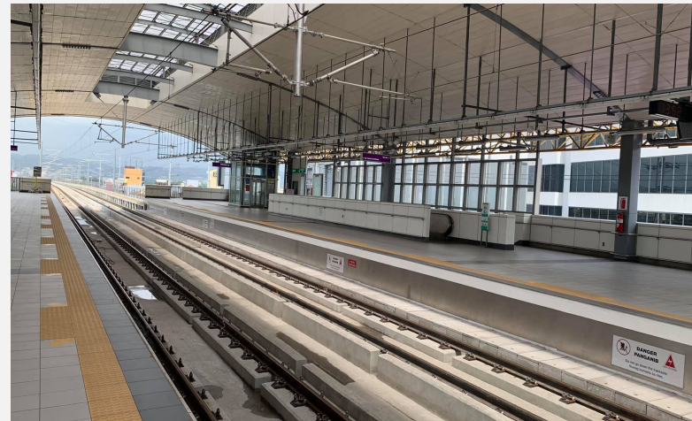
LRT 2 East Extension
